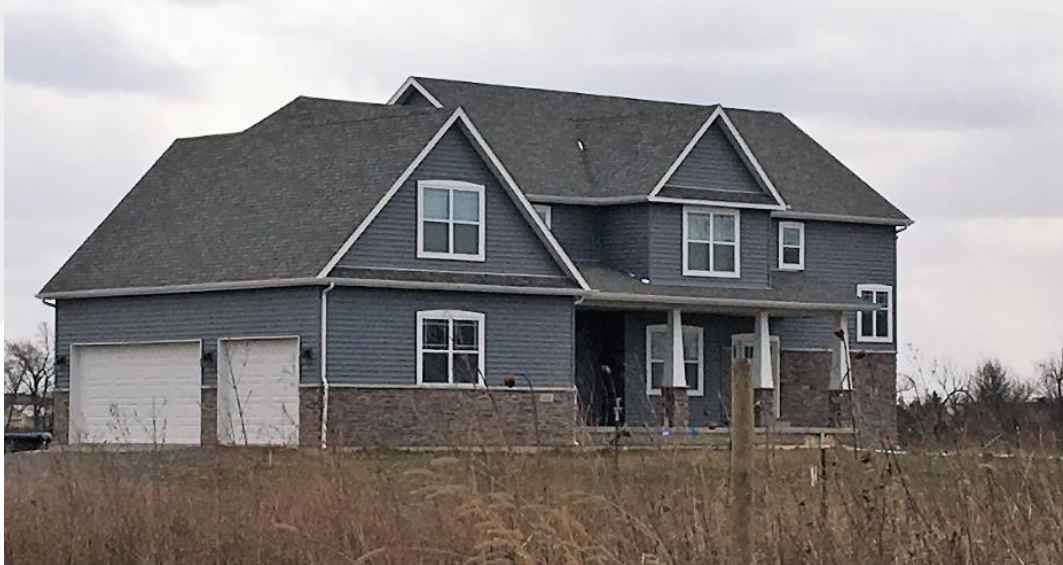
4,255 square foot estate home under construction, adjacent to Portage Solar Farm (Solar Farm 2)
