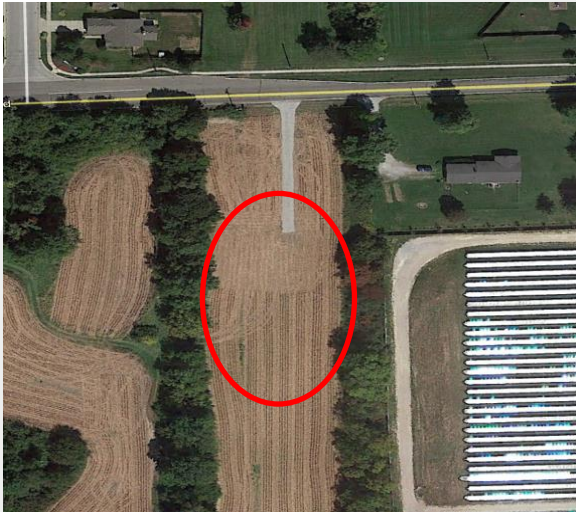
Dominion Indy III Solar Farm (Solar Farm 4) September 2014
